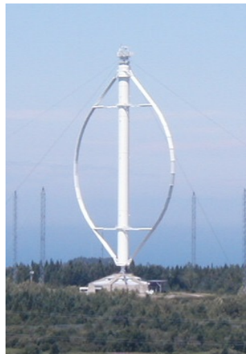
Figure 1.2: An example of a large VAWT (Darrieus wind turbine). Source: Guillom [2005].
