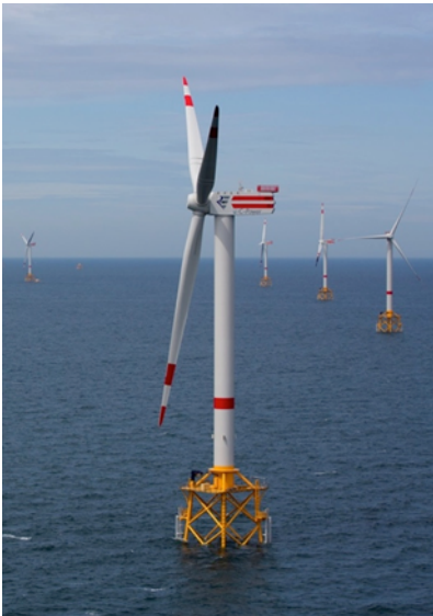
Figure 1.7: Wind turbine on jacket foundation. Source: AVRГ-VUB.
