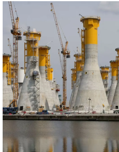
Figure 1.8: Gravity foundations under construction in France. Source: Lewis [2022]
