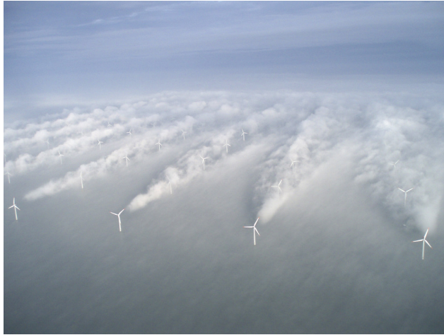
Figure 1.4: Wake effect – Turbulent wind flow generated behind each turbine in the Horns Rev wind farm in Denmark [Christian Steiness/Vattenfall/Flickr, 2010].
